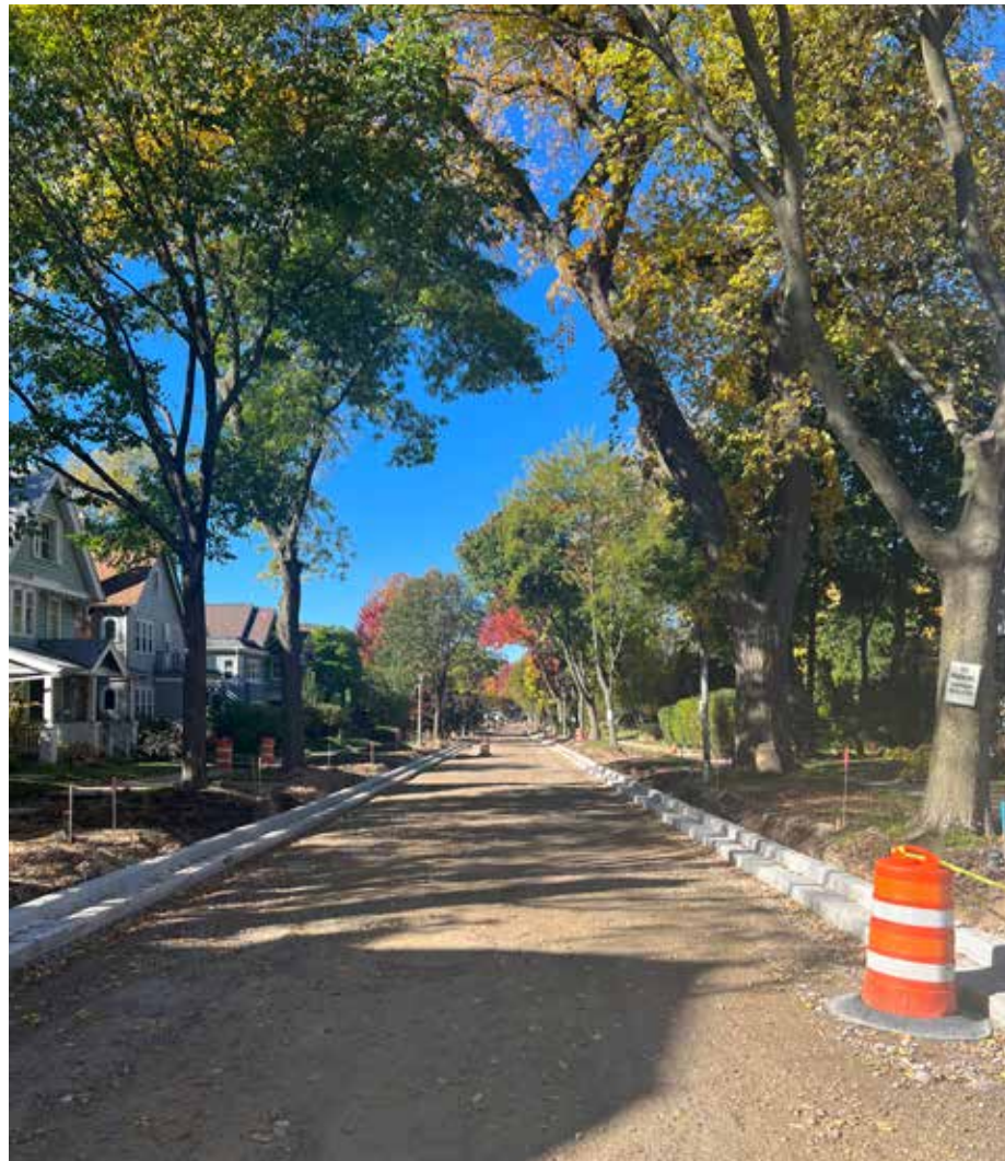
East Stratford Court, pictured looking west, has been under construction since April 2023. New curb and gutter was installed in the fall, and the road was recently paved.
