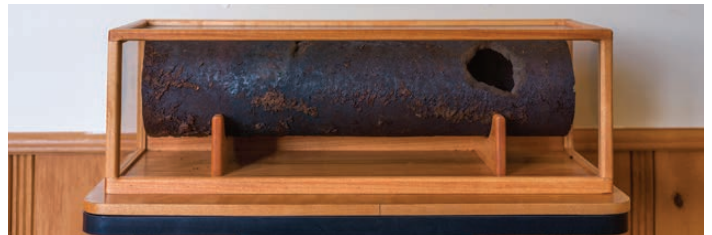
This worn-out lead pipe on display in Village Hall shows the condition of many local water mains.
