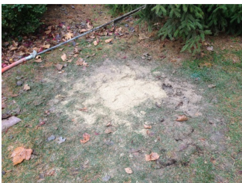
Lateral lining completed; awaiting topsoil and seed.
