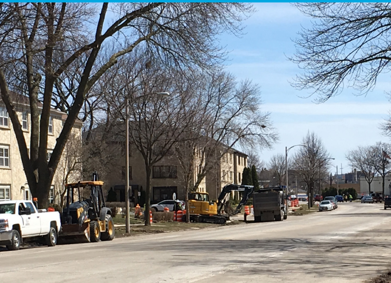
↑ WE Energies excavates along the sidewalk for the new gas main installation.
