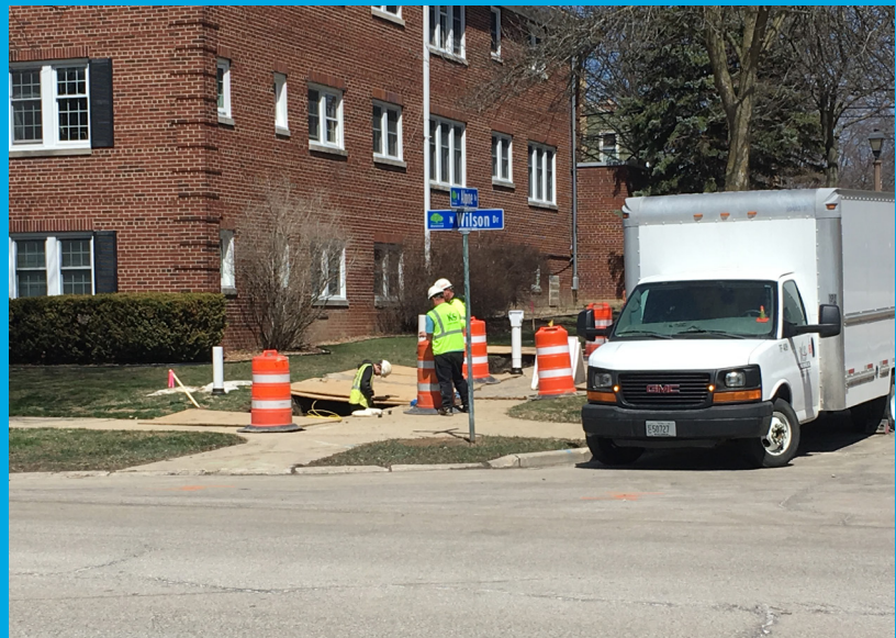
↑ KS Energy Services excavates along the sidewalk for new utility installation.
