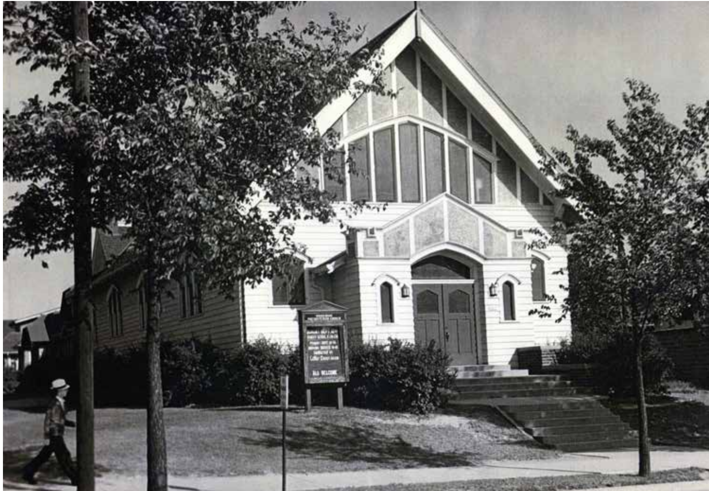
The "little white church" was the North Shore Presbyterian congregation's first home. After the congregation moved, several businesses occupied the building until it was demolished in 2018 and replaced by North Shore Bank.
