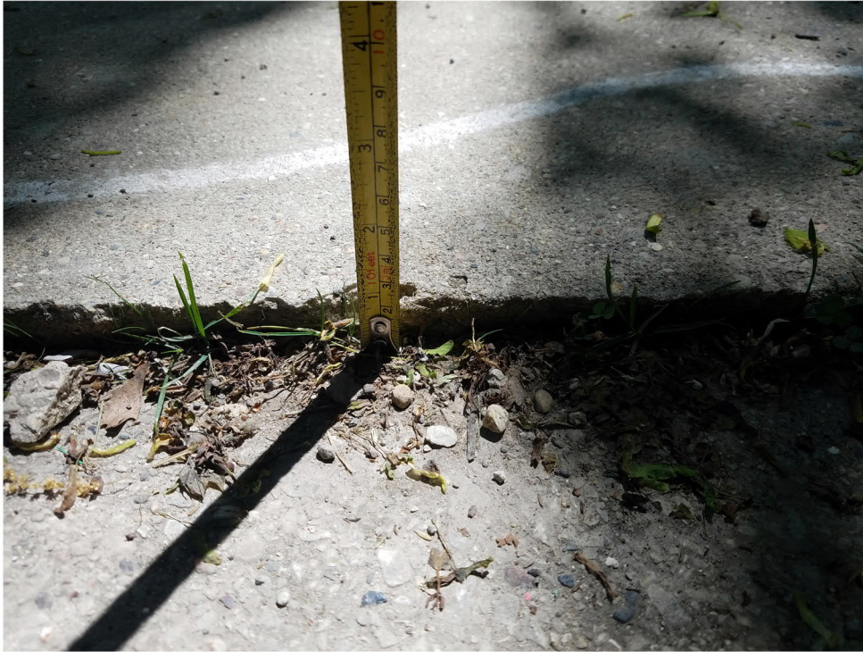
Criteria 4 - 3/4-inch Differential Settlement
