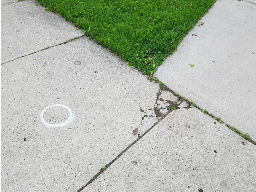
Criteria 6 - Fractured into Several Pieces
