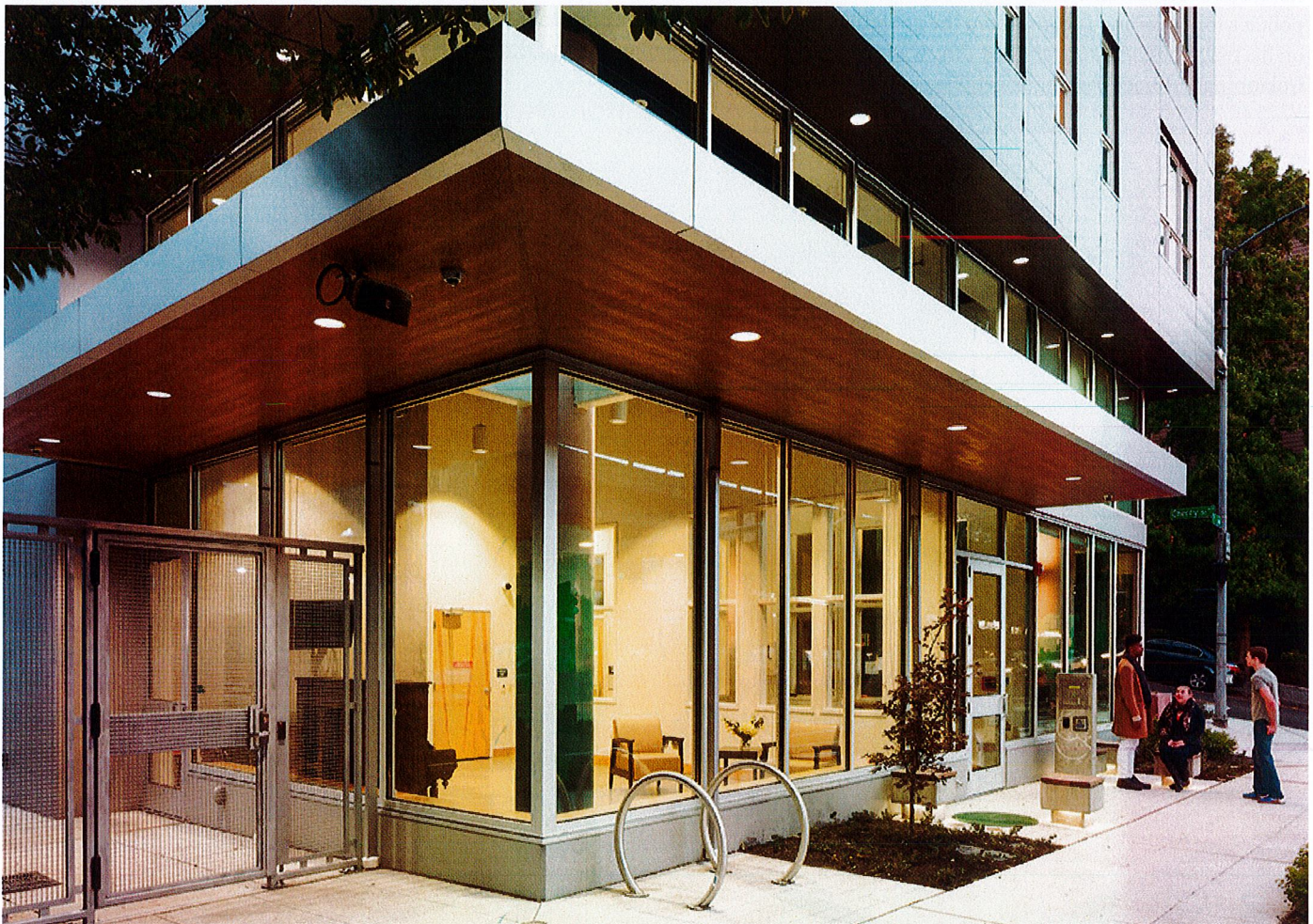
Carless in Seattle: Plymouth on First Hill's apartments are now home to some of the city's formerly homeless disabled population. Photo courtesy SMR Architects and Plymouth Housing Group.
