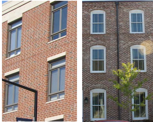
Figure 535-23-10. Vertically Oriented Window & Exposed Lintels
