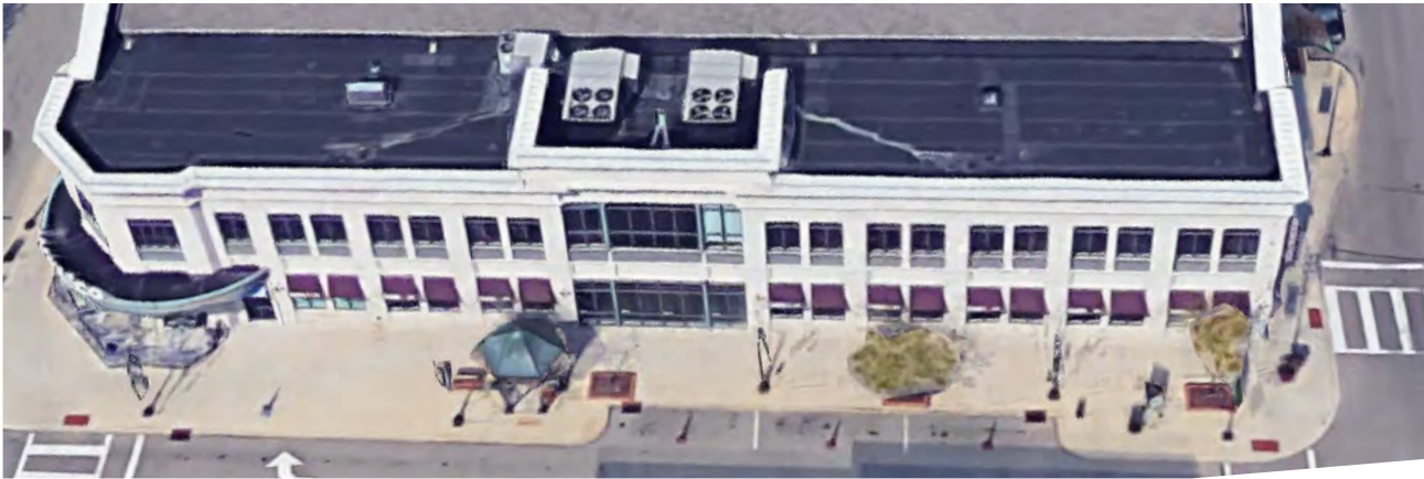
Figure 535-23-18. Rooftop Utilities Screened from the Public Way by a Parapet
