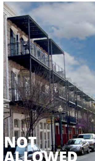
Balconies: Covers More than Allowed Facade Area
