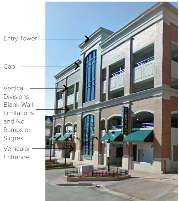
Figure 535-23-17. Example of a Parking Facade
