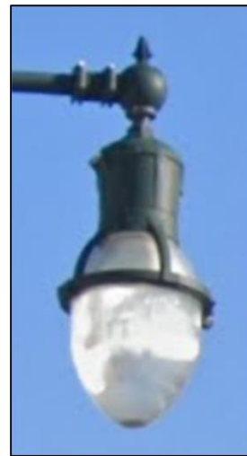
Figure 4 Holophane Atlanta and Memphis Teardrop Fixtures Used Along East Capitol Drive and North Oakland Avenue
