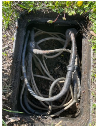
Existing splice. Submersible Terminal Blocks are recommended for all handhole splices
