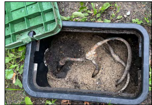
Existing Pull Box
