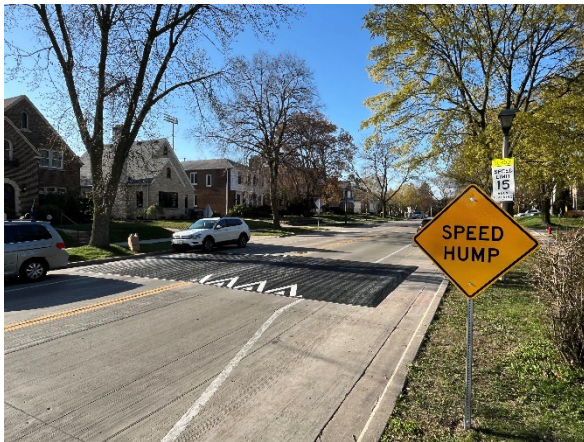
Temporary Speed Table: N. Morris Blvd. (north of E. Pinedale Ct.)
