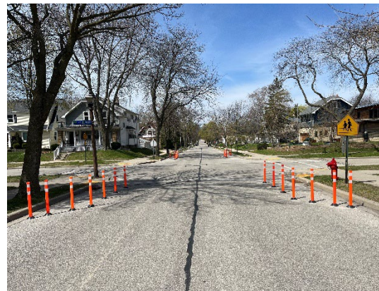
Temporary Curb Extensions: E. Kensington Blvd. and N. Larkin St.
