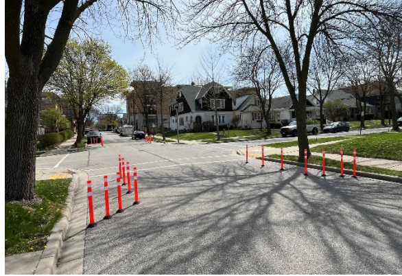
Temporary Curb Extensions: E. Kensington Blvd. and N. Bartlett Ave.
