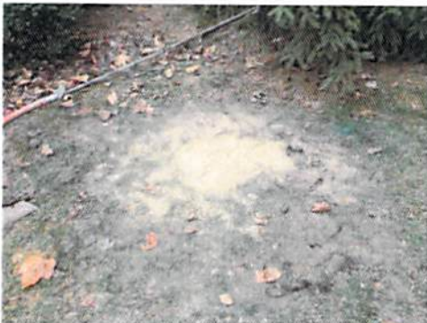
Lateral lining completed; awaiting topsoil and seed.
